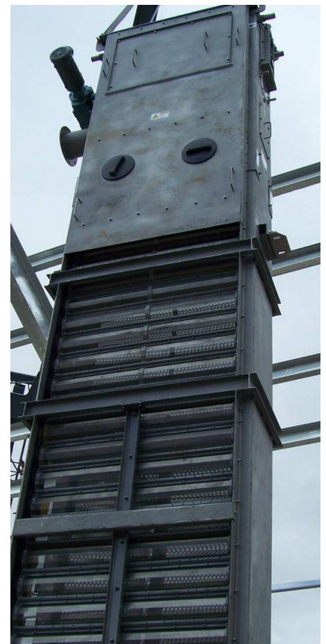
Installation of Eliminator Band Screen by crane.
